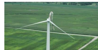
Wind Blade Damage by Heavy Storm
